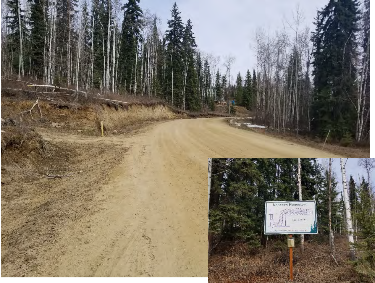
Figure 21: Haman Road constructed, looking north from Roland Road. Inset: the Koponen Homestead subdivision, through which Haman Road was developed. Source: PDC Engineers.
